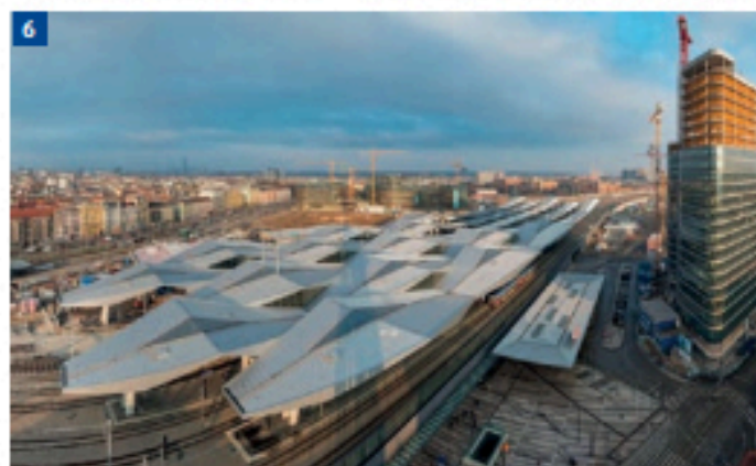
Vienna Railway Station, Austria (Foto 4: © ÖBB Raman Bänisch, foto 5, 6: © Renée Del Missier, Unger Steel Group)
