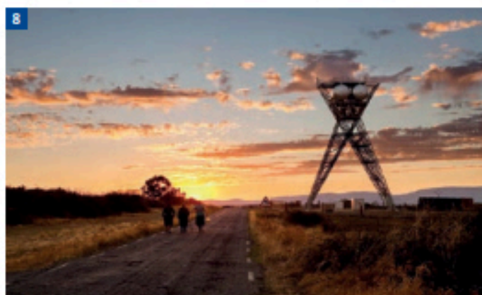
Water Tank, Guijo De Coria, Spain (Foto 8: Lluís Casals)
